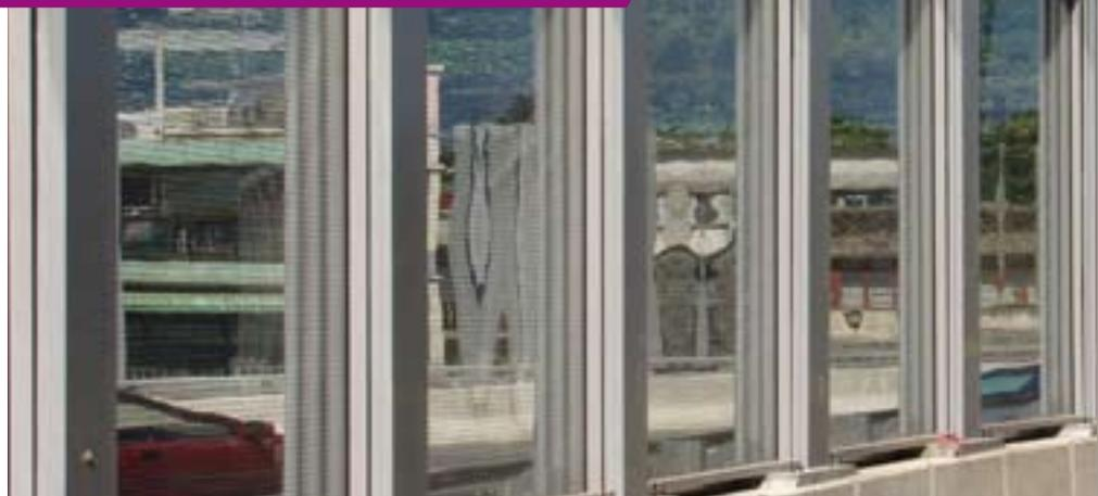
**Large-size, highly transparent extruded noise barrier sheets with integrated bird protection.**
