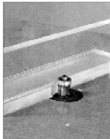
Fig. 21: Milling down beads of adhesive
